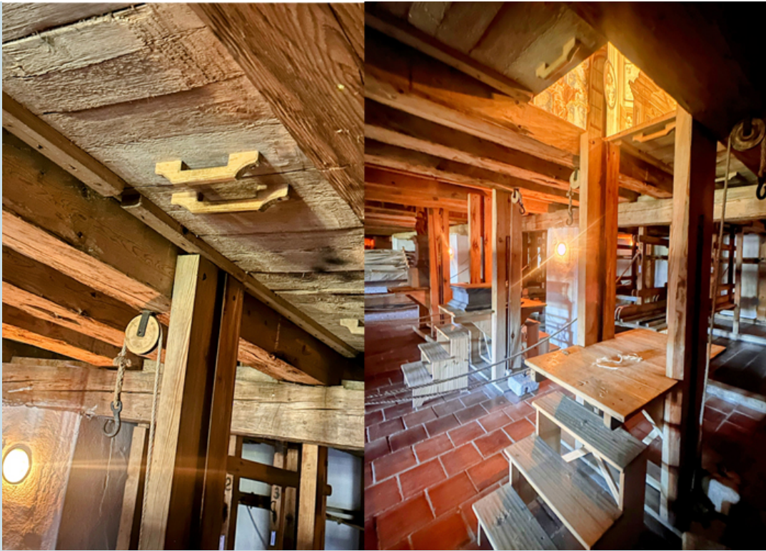
Detail of the trap door – closed on the left and open to the stage on the right. Photo courtesy of Kiara Pipino.
